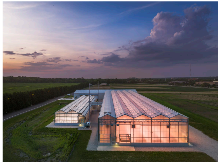
Figure 3. Controlled Environment Agriculture Research Complex (CEARC) at the Ohio State University. Two glazing materials (glass and ETFE) are used for Venlo-style greenhouses. (Photo credit: Brad Feinknopf)
