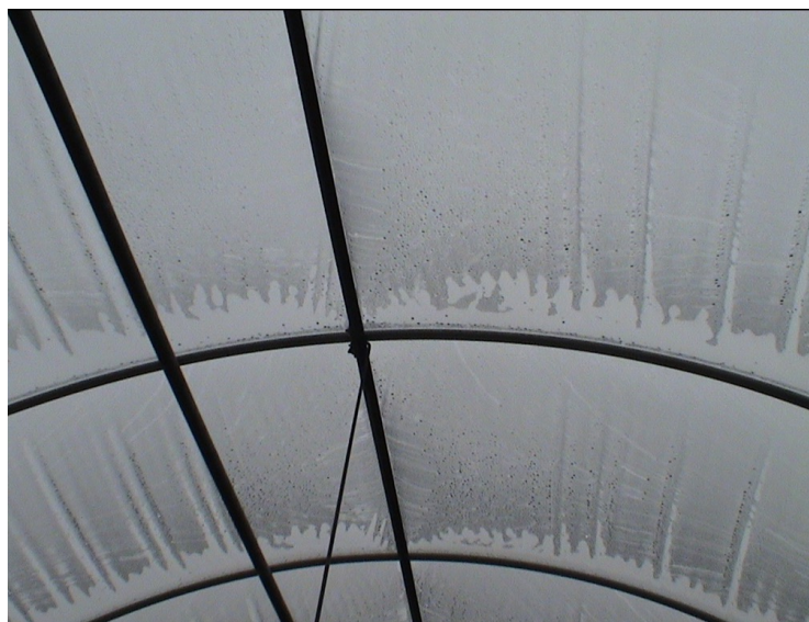
Figure 2. Condensation observed on the surface of polyethylene film glazing covering over an arc-roof greenhouse (Photo credit: Dr. Peter Ling, Ohio State University).
