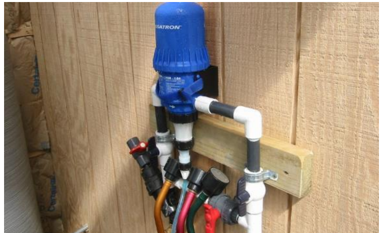
Figure 2: Many growers use only a single injector when dealing with water quality issues in the greenhouse. Over time some of the integral parts of the injector become worn. (Photo by Tom Ford, Penn State Extension)
